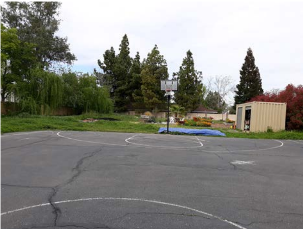
Looking north at west side of parking
