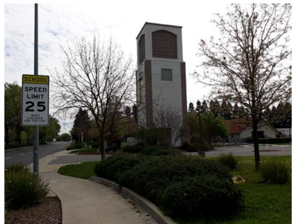
Tower building fronting Bruceville Road
