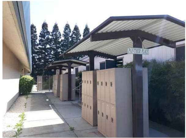
Covered walk and lockers
