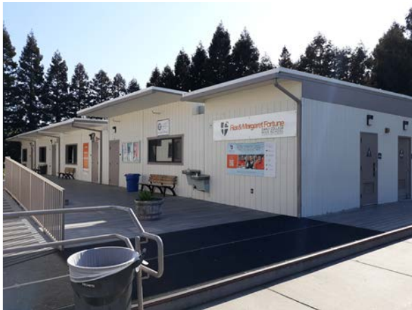
Southwest view of the west classrooms
